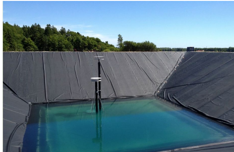
Pit TES in Dronninglund (source: PlanEnergi, 2017).
