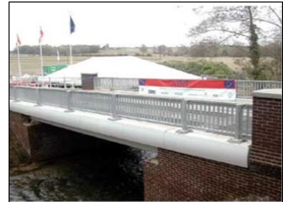
West Mill Bridge, England, 2002 ( First Composite bridge in Europe)
