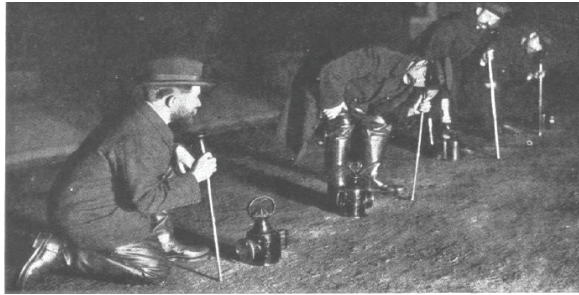
Figure 3. Nearly 100 years ago, night crews listen for water leaks using stethoscopes and aquaphones.
